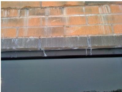
Mortar or masonry run-off onto anodized window frame
