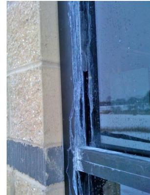
Mortar run-off onto anodized window frame
